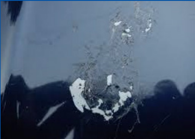
+ BAT DROPPINGS STAINS
